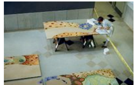
Panels in progress on site
