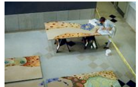
Panels in progress on site
